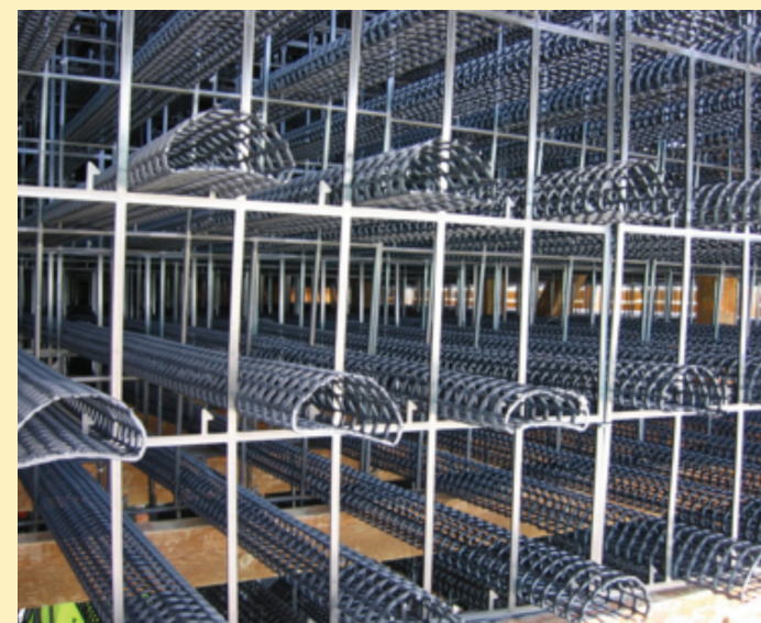
New fill media (Left) and drift eliminator (Right).
