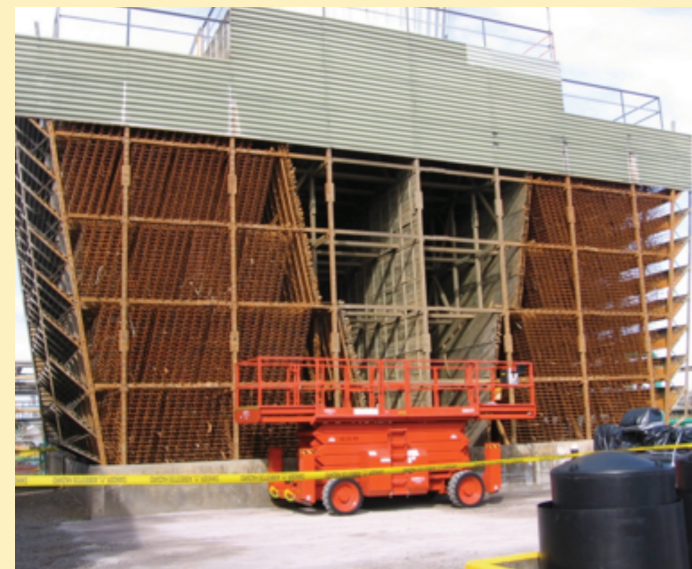
West Cooling Tower during refurbishment (before and after).
