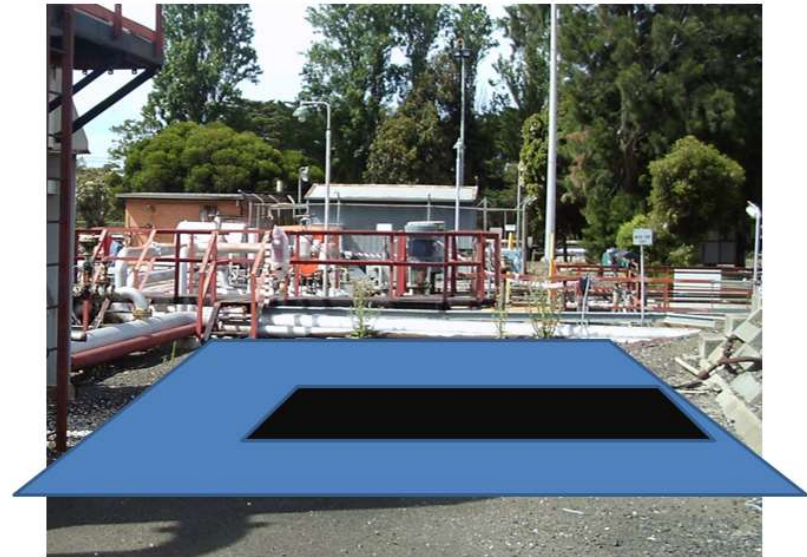
AC filter skid location on new concrete pad.
