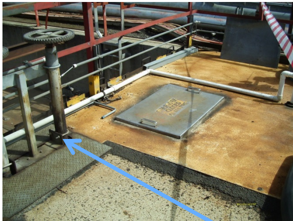
Gaps around handwheel penetrations sealed
